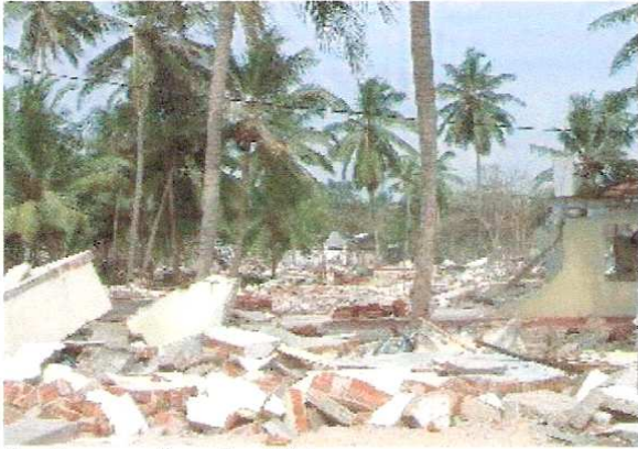
The Damage – December 2004
